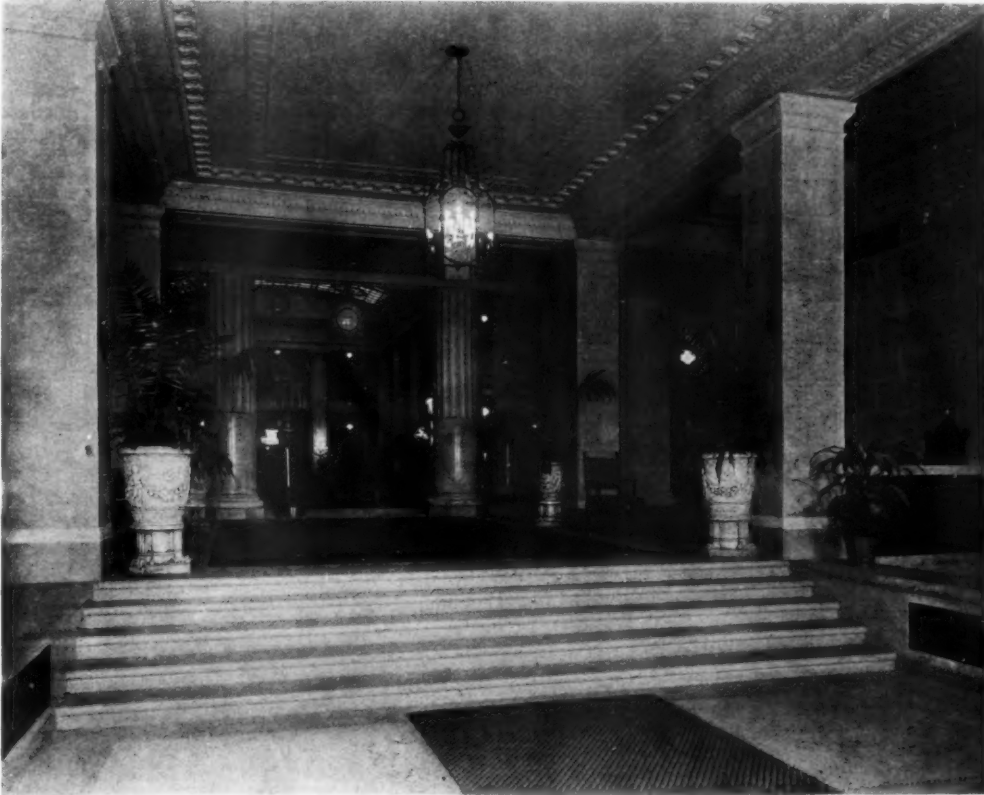
MAIN ENTRANCE LOBBY
